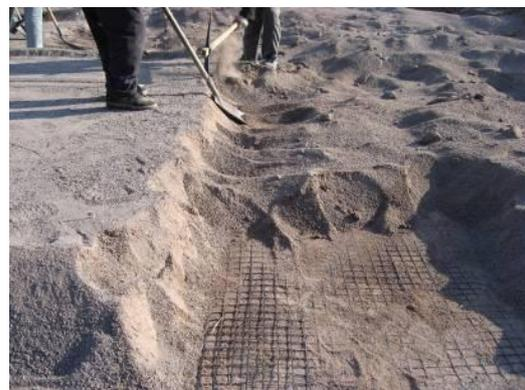
Differing grades of E'GRID and Triax geogrids were installed as if they were being used in construction of a carriageway with the 3 different rock fills. They were then excavated and their strengths were measured and recorded relative to their original properties.
